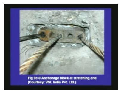
After the stretching of the tendons, you can notice that they have anchored in the anchorage block. You can see the wedges that are holding the tendons in place and this anchorage block is transferring the prestress from the tendons to the concrete.
