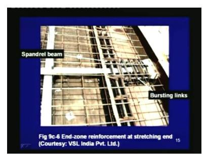
This photograph shows the end-zone reinforcement at the anchorage end of the prestressing tendons. Bursting links are provided to resist the stress concentration that is generated after the prestressing operation. Also note the spandrel beam which runs along the edge of the slab and this spandrel beam is designed for torsion. Hence, the links of the stirrups that are provided in the span-beam are closed. That means there is a complete circulatory for torsion in the spandrel beams.
