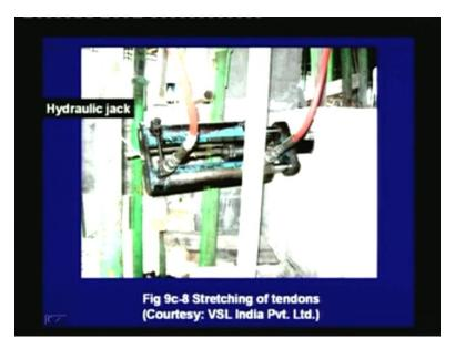
Once the concrete is caused and it attains a desired strength then, the slab is posttensioned by hydraulic jacks. In this photograph, you can see that the hydraulic jack has been placed at the side of the slab and the tendons are being stretched by this jack to the required amount of prestressing force
