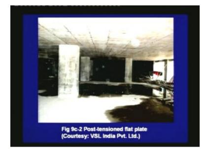
In this photograph, we can see a post tensioned flat plate after construction. We can notice that there are no column capitals or drop panels and see that the bottom of the slab
