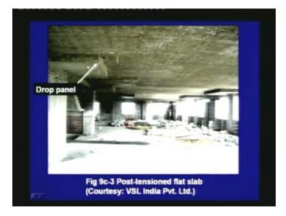
In this figure, we can see a post tensioned flat slab where there is a drop panel. You can see that the slab has been thickened around the columns and in other columns also, you can notice the drop panel. Here also for most of the areas, the bottom surface of the slab is flat and hence, this type of construction also creates much less obstructions to the service conduits.
