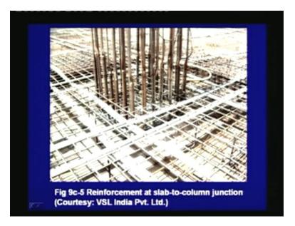
This is a closer view of the reinforcement around the slab-to-column junction. You can see that ducts have been spaced closely around the columns and also the reinforcement is much higher around the slab-to-column junction which helps to transfer the shear that generates in this junction.
