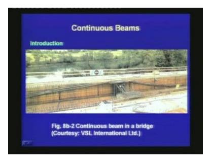
This is a photograph of a continuous beam in a bridge and here you observe that at the support region, the tendons have been brought up and again after the support region they go down. In a continuous beam, the cable profile is very important. Hence, attention should be given to have appropriate cable profile in the span region as well as in the support region. Next, we shall study the analysis of continuous beams.
