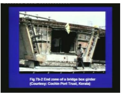
This is another photograph of a bridge box girder. Here, you see that the anchorage blocks have been placed at the end zone. This creates substantial amount of stresses in the end zone and the strands develop the prestress at the anchorage block itself.
