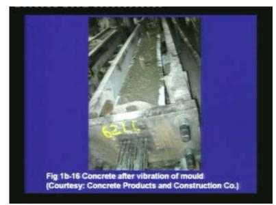
After the concrete is dropped, it is vibrated. In this case, the mould itself is vibrated. There is some vibration done by needle vibrators so as to make sure that the concrete is well compacted without voids. After that, the finishing is done properly to make sure that it is a smooth finish at the top after the concrete has been cast.
