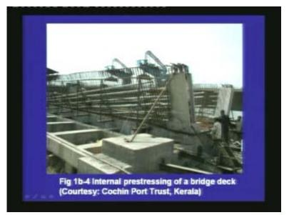
In this photograph, we can see that the tendons are located inside the member. Once the concrete is cast, these ducts and the tendons will be concealed by the concrete and it cannot be seen from the outside. Thus, internal prestressing is different from external prestressing based on the location of the tendon with respect to the concrete.
