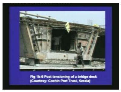
This photograph shows a post-tensioned box girder bridge. Here we can see that some of the tendons have been stretched. It has been fixed by the anchor blocks, and thus some prestress has been applied to the sections. (Refer Time Slide: 23:57)
