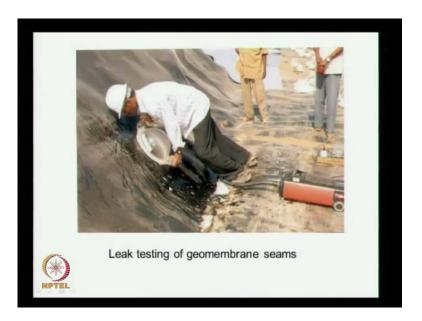
It should be a tested by some suitable means and here we see this this person doing the leak testing by blowing some air or the sop solution. There is an ASTM requirement that any pressure that is applied, it should be maintain a constant for certain duration of time and if it is not so then the seam has to be redone.
