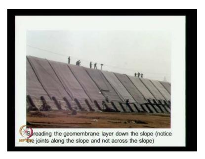
Here, you see another picture of these this spreading of the geomembranes and you see that all these joints they are given along the length of the slope, and not across the length across the slope because the gravity force is acting down. If we provide a joint along this in this direction, it is subjected to lot of tensile force and it might rupture in the process of the service life.
