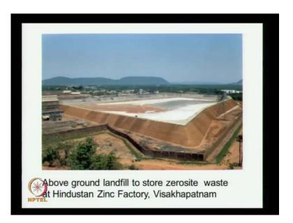
I will very briefly explain the construction of the one of the first landfills in India, this picture that you are seeing is the landfill that was constructed at the Hindustan Zinc factory in Visakhapatnam. This is to store the zerosite waste that was produced as part of the zinc smelting process and this particular factory has been in operation right form 1950s. So, they have accumulated lot of zerosite which is a highly toxic waste and that needs to be safely disposed off.
