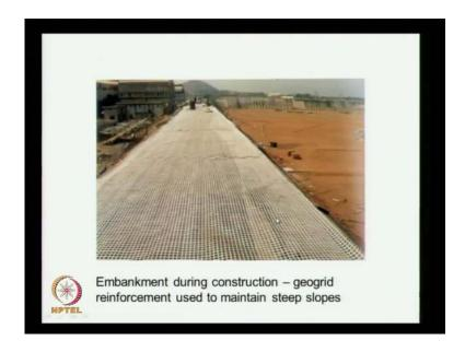
Here, we see the construction of this of this embankment using the some geogrids.
