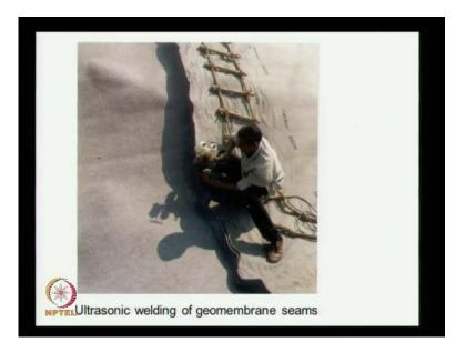
Here, we see the ultrasonic welding of the joint the joints at the geomembrane over lap locations, whatever joint that is produced.
