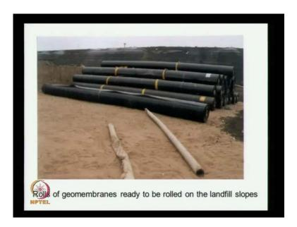
Here, we see this geomembranes and these geomembranes they should be at least 5 meters long, so that the requirement for the joints is lesser.
