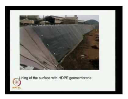
Here, we see the picture of the geomembrane that is laid on top of this of the slope that is constructed.
