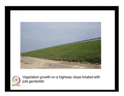
And here we see an example of the vegetation growth after covering this area with a jute geotextile.
