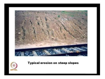
And some example applications are shown here. This is a typical scene on most of the highway and the railway embankments because of the flow of the rain water, we have lot of gullies formed mainly because there is nothing to hold the soil together. If there is good vegetation, the roots of the vegetation can hold the soil together and prevent the erosion.
