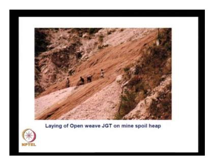
And here we see the application of jute geotextile being spread on a spoil heap mine dump to promote the growth of vegetation.
