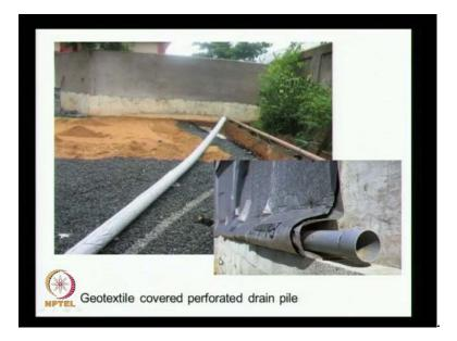
Here is another example on how we can utilize perforated pipe. Here we see a perforated pipe covered with a geotextile. And here you see another close up, we have this PVC pipe with perforations. We need to cover it with some geotextile so that this pipe does not get fill with fine soil particles or wet clogged. Once these are fabricated, they can be laid along the drains at some depth, to provide path for water that enters the pavement that to escape from out of the soil structure.
