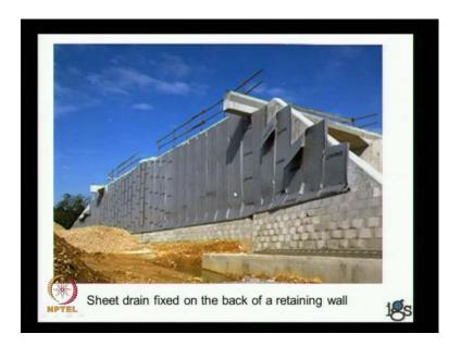
And here we see the application of a sheet drain or a boat drain, that can be fixed on a retaining wall like this. This soil is compacted behind it and any water that enters the back fill can go through this, the geotextile then come down. And here you see a perforated pipe that is collecting all the water, that comes down these drainage boards and it is safely led away from the structure.
