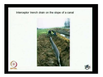
And here we see the application of a geosynthetic trench drain. This is to provide or to trap any water that comes through say for example, there is a canal here and if you provide this interceptor drain, this water cannot or will not flow into the surrounding. And if you provide these drains on a side slope or on hill slopes, we can catch the water that enters the ground and safely lead it away from the critical points.
