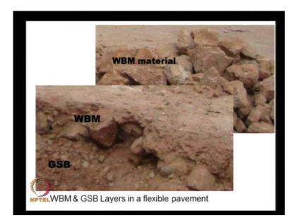
And here we see some examples of these base course materials, this is the WBM water bound macadam. Actually these are very large size stones and here you see the trisection of a flexible pavement with a very large size stone that are bound together by using a some granully soil, morrum soil. And below this we see this GSB that is the granular sub base and both the WBM and the GSB layers, they are usually highly porous so that they also act as drainage layers in our pavements.
