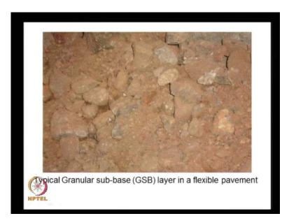
And here you see this, the close up of the granular sub base layer, which is consisting of the smaller sized particles as compared to the base course.
