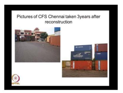
And after these repairs by using geocells, geotextile as a separator and geocells as a surface confinement layer, this the performance is actually this entire yard it has maintained a good level. This is pictures taken three years after the reconstruction, and here you see that there is a very good support that is given to these containers.
