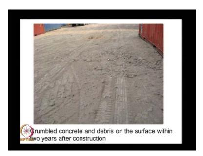
And there is another thing, basically even in a reinforce concrete pavement what we see within a very short time is the crumbled concrete, and debris flying all over because these operations they apply very heavy load. And the sometimes with impact load because when these vehicles move by carrying these heavy containers, they exert lot of pressure on the foundation soil.
