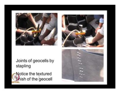
And here you see this welding of the geocells because these geocells they typically come in a width of 3 to 4 meters and 20 meters length. And when we are spreading very large length, we need to join them together. Here we see this stapler that is joining this geocells, here you see this stapled geocell. The particular geocell that was used in Mumbai, it was a textured on. And there are no openings, there are no pocket openings in these geocells.
