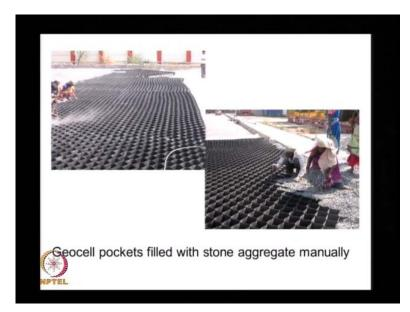
They are manually spread and anchored by using some wedges. And then they are filled with stones ships and then they are compacted.
