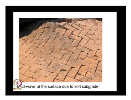
So, this is the scenario just about seasons after this container yard was thrown open for operations, at the ground surface the mud wave got reflected and the entire surface got angulated like this. And this is a typical failure that is attributed due to the formation of the mud wave. Just like how the surface waves form in the ocean similar thing happens even in the soft clays get and that got reflected.
