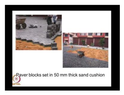
And here you see this sand in sand cushion and then the paver blocks. This particular paver block arrangement is called as the herring bone. And they are very well interlocked, that interlocking is essentials because these vehicle that move within the container yards, they have a very heavy rubber tires that produce lot of surface friction. And unless these are very well interlocked these tiles might just simply come loose.
