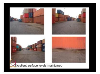
And here you see some more pictures of the same thing. This entire stretch was the same 1 that you have seen earlier with lot of mud waves that were formed. And now because of the confinement that is given at the surface. And then a geotextile reinforcement that is given at some depth the pavement has adequate stiffness. And then the drainage was also provided because at some depth we have a trap to collect the water, and lead it safely away from the away from the yard.
