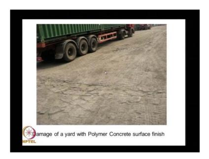
And here you see all these rutting, and this particular thing is with polymer concrete surface finish on top of the reinforced concrete.
