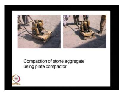
And the top surface was finished by providing the sand dust and then compact with a plate compactor.
