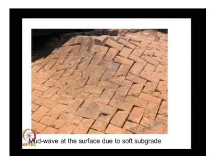
This is a typical failure that we can expect whenever there is no surface confinement. And if they if we are able to provide a very good confinement at the ground surface, where the pressure are very low we can have better performance.
