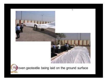
Here you see the geotextile that is being laid on top of the WBM. And here you see this the geocells being spread and these geocells.
