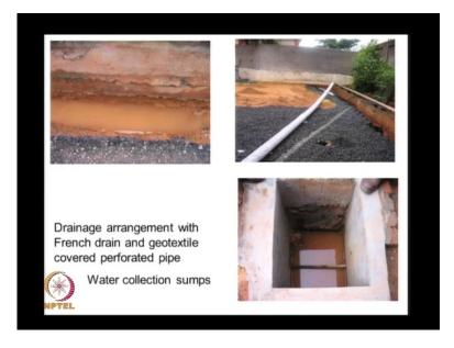
And here you see this the peripheral terns, and then below there is French drain like this. This is actually it is a perforated pipe covered with a geotextile. And this is provided at some at depth and then the water is lead into some traps, or some sumps at periodic intervals. And in the heavy monsoon rains we just simply put a pump and pump out the water. So, that we do not have much of water stagnation.
