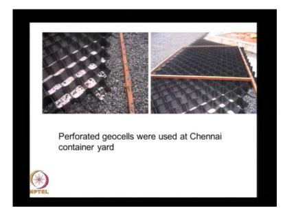
And here you see this construction, the geocell that is used it has open apertures. So, that there is facility for cross draining in addition to this strength that we have.
