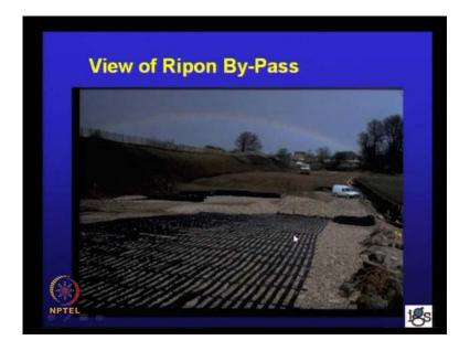
Basically, we have number of these this polymeric strips, each may be about 50 kilo Newton to 100 kilo Newton capacity, they all are linked together.
