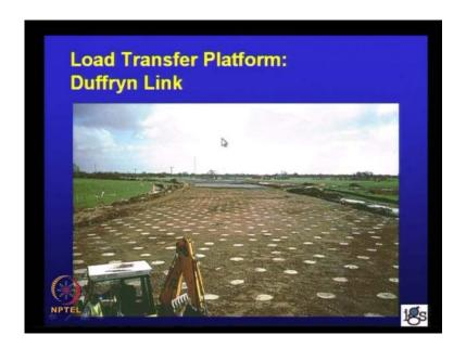
And another place where, these low transfer platforms have been successfully, used was in the duffryn link, once again we see this a small diameter piles that are pre-cost and pushed into the ground.
