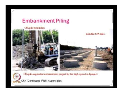
And let us see some of the examples here at one project, we see the castings to piles, we which are, which we call as a castings to piles or continuous flight auger. And on the left hand side, we see the bore well being made the right hand side the finished piles that are already in place.
