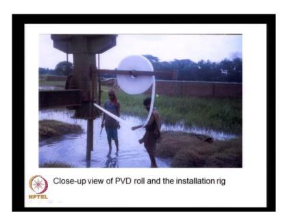
Another close up of this same thing is, actually we take the PVD's from this roll and feed it into this rig, and connected to the anchor plate.
