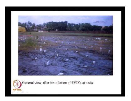
Here, we can see the view of this site that is treated with a pre fabricated vertical drains. We have number of these and after the PVD's are installed, we need to lay the blanket soil that is highly permeable, so that all the water that comes out or can travel away from construction site.
