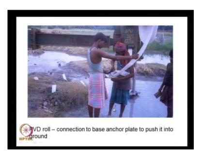
Here, we see an example of the PVD, that is coming in a roll and this PVD is being connected to anchor plate, that gets that is connected to this rod. This simply pushes the anchor plate and along with the anchor plate the PVD enters the ground. Here, we can see some PVD's that are already installed and the entire field is a soft clay soil.
