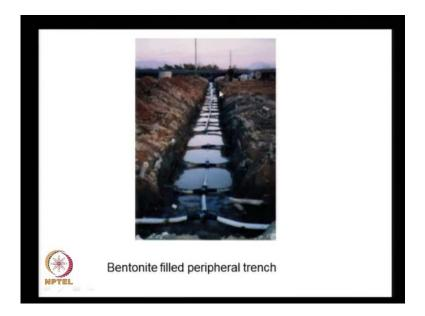
Here, we can see the bentonite filled trench around the treated area.
