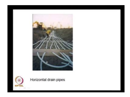
Here, in this photograph, you can see these horizontal pipelines that are laid on the ground surface.
