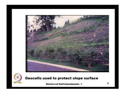
Here is an example on the face treatment using combination of geocells that we have seen earlier, and and then the vegetation that is growing through the through the pockets of these geocells.
