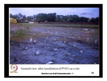
Here you can see the ground treated with p v d's, then on top of this once we apply the surcharge load either an embankment or our foundation the soil quickly consolidates, and during the construction time itself we can achieve the all the settlements.
