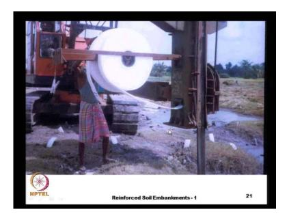
Here we see the instillation of a pre-fabricated vertical drain is actually it comes in narrow strips of about 100 m m wide, and 2 to 3 millimeters thick, and this comes in length of about 100 meters, and here we can see these p v d's installed it one site.
