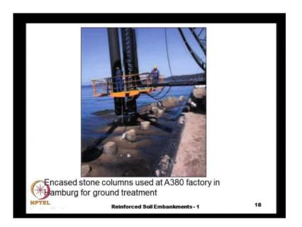
Here we see an example of an encased stone column, where in we have a granular column, but that is placed inside that cube of geotextile or geogrid. So, that a combination of this granular material that is encased within the geosynthetic behaves like a very strong and stiff column this, we will we will see in the some other lecture and the particular photograph that you have seen this is the ground treatment that was given to the A 380 factory in hamburg Germany.
