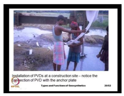
And here, we see the application of pre-fabricated vertical drains at a construction site with a very soft clay subgrade, soft clay foundation soil and here we see some P V D's that are already installed. And here, we see these 2 people attaching the P V D to an anchor plate.
