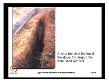
And this is how, we anchor the rope net top of the slope is actually, there is a 1 meter deep trenches and which is 0.5 meters wide. And it is the rope net is anchored in the trenches and the size of trench, especially the depth of the trench. And the width, they are decided based on the amount of tension, that is likely to be developed based on the size
