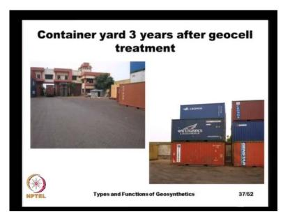
And this constructed surface is actually, it is absolutely flat and these the photographs taken 3 years after the geocell treatment of the same area where, we have seen these mud waves, that were formed. And is actually, the entire yard is flat and the that allows the free movement of the of these container vehicles and another problem with the uneven ground is if these containers, they are stacked on uneven ground, they tend to get
