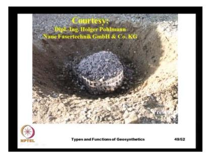
And here, we see an encased stone column using a geogrid is actually when geogrids can be used, because they have very high tensile strength and they can provide very good confinement and in areas where, we do not anticipate any contamination of the stone column material by the soft clays, we can use a geogrid.
