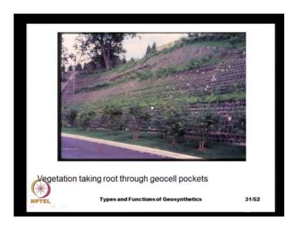
And here, we see the construction of a very steep slope using geocells and the and because of the open geocell pockets, we can promote the vegetation through this open pockets. And once these the vegetation takes root the entire thing could be a green color surface and we will not even see the that the geocells are applied for construction of the slope.
