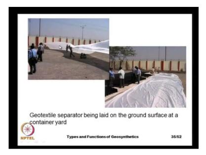
And here, we see the construction process, first we layer of geotextile, that can act as a separator.
