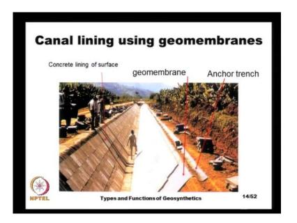
And here, we see the application of a geomembrane for canal lining and here, we see this the geomembrane, that is lined on the canal and the geomembrane itself is protected by concrete panels on the top. So, that the geomembrane is not directly exposed to the sun, because all these polymeric products, they have they get degraded, because of the exposure to light and the heat that is the sun. And the geomembrane, that is lined up, that is anchored at the top use using an anchor trench.
