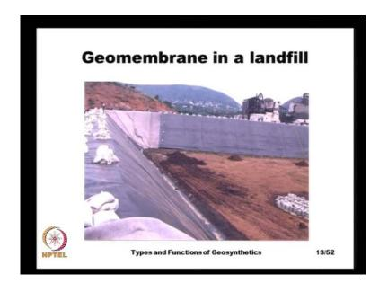
And here, we see the lining of a land fill with a geomembrane the main purpose is if there is a hassudust waste or a toxic waste the this the product of this toxic waste, they will not flow through the landfill and contaminate the ground water.
