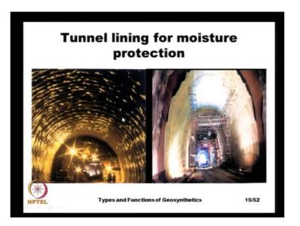
And here, we see the application of a geomembrane for canal lining to prevent the moisture from seeping into the inside of the tunnel.
