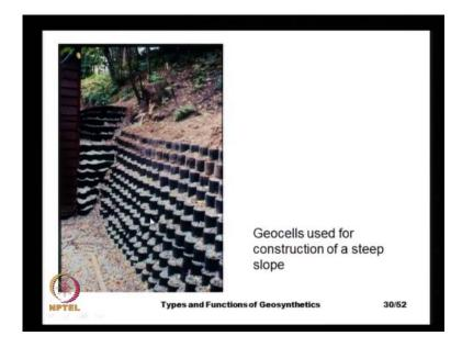
And here we see the application of a geocell for construction of a steep slope or for stabilizing the steep slope.
