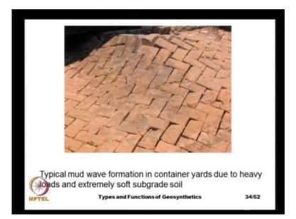
In fact, this particular container yard in Chennai was built on reclaimed land and the thickness of the soil, that is placed is about 1 and half 2 meters very very thick soil layer was placed and then that was stabilized by good compaction. And then on top of that there was about 500 millimeters thick pavement layer in the form of boulders then aggregates and then sand cement mix and so on.
