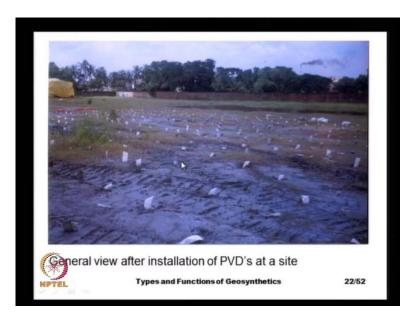
And once the entire ground is treated with pre-fabricated vertical drains, we can apply some surcharge on this and the soil. And the amount of surcharge that, we apply should be corresponding to the expected foundation pressures that, we have after the full construction takes place.
