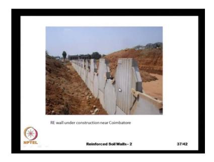
And here we another farm that we can have for the facing panels here, it is a bit of hexagon shaped facing panels, once again with vertical grooves and without much of an architectural finish. And this is part of a an approach road for a fly over, that is under construction here we can see this the bridge deck is going to come out this level, and this is all the length of the retaining wall.
