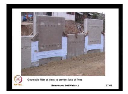
Here, we see another detail of the of this facing panels, and apart from the stone aggregate that we have because the joints they are much wider in these facing panels. We give some geo textile cover, so that they act like a filter to prevent any fine soil particles from coming out of the back fill, and here they are glued together, so that they are in position. And once the soil is placed behind and are compacted, there is no need for any other support the geo textile will be in place.
