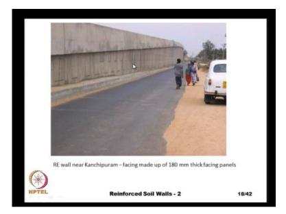
And another popular method of construction is in India is using concrete panels, which are much wider and much taller, and these this particular flyover is also built near to Chennai in Kanchipuram and the facing is made up of one 80 mm thick facing panels.
