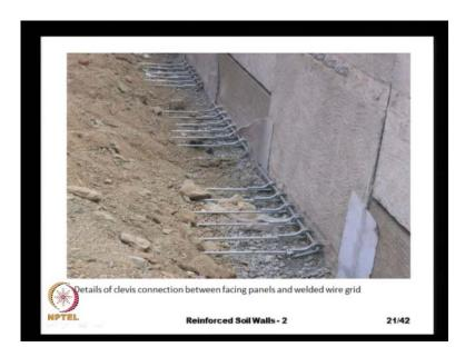
And here we see a detail on the connection we have the panel facing panels and this is the welded wire mesh reinforcement, and on the front side we connect the reinforcement by means of a cross bar. And this cross bar is a 16 millimeters diameter and these hooks they are anywhere from 9 mm hooks to 12 millimeters depending on the company, different companies use different grade of steel and different diameters.
