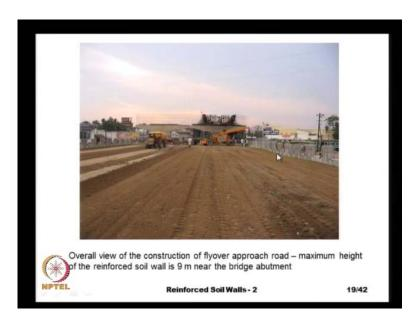
And here you see one approach road, that is under construction this is for a level crossing, the bridge deck is going to come up at this level and this height is nearly 9 to 9 and half meters. So, the approach road is going to come, and then that is on both sides this approach road is vertically supported by reinforce soil retaining walls. And here you can see this, the crane that is handling the facing panels and this lorry is watering the soil.
