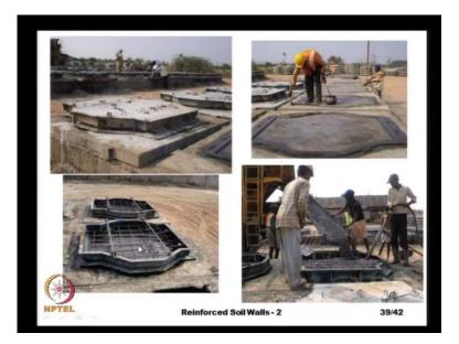
Here, we see these blocks under manufacture is actually this before we do anything on the mould we apply some oil, and then we put in the nominal reinforcement that is required for withstanding the handling stresses. Then we have we pour the concrete then with after the concrete is set, we can de mould them, and then take to the site, and here you can see these hooks in place that are used for connecting the reinforcement element to the facing panels through the cross rod.
