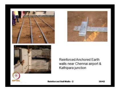
As I mentioned earlier we also use reinforced earth tankers and in this case when we have the steel strips like this one here, this particular retain wall is built in Chennai on the highway leading from IIT Madras to the airport. This particular steel strips they are 50 mm wide and thickness is 6 millimeters and as we discussed earlier the reinforced force is mobilized through skin friction.
