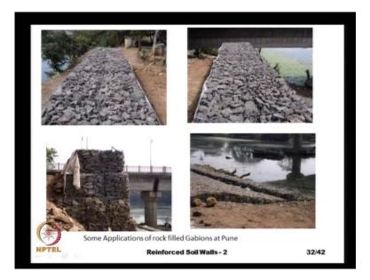
Here we see the application of the gabions, gabions are either steel wire baskets or polymeric rope net baskets, here we have this steel wire baskets, and this particular wall was built as a river training work. And the entire retaining wall was built using wire baskets filled with stone aggregate and this was built in the city of Pune, as a river training work and there was no reinforcement given.
