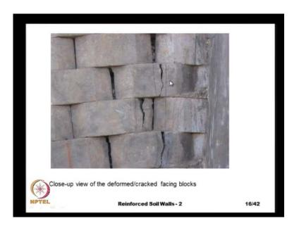
And here is the close up of the cracked blocks and not only the cracking, but the gap between some of these these blocks it has widened, and because the aggregate layer is placed just behind this modular blocks nothing has happened. If it was just a plain soil behind this modular blocks, the soil would have started coming out, but because large sized aggregate particles were used nothing has happened.
