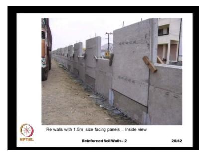
So, that this soil can be compacted and here we see the close up view of the retaining wall the with the facing panels, and the when this facing panel is cast we provide some hooks. So, that the reinforcement layers can be connected, and the size of each of these panels is 1.5 meters by 1.5 meters and the thickness is 180 mm, so the weight of each of these panels is about nearly one ton, so we require some light cranes to handle these panels they cannot be handled by normal people.
