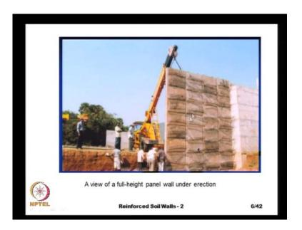
Well, as I mentioned the full height panel walls the advantage is there is no assembly required of individual modular blocks or the individual panels and when the height is limited to about 3 to maximum 5 meters. We just simply crust one full height panel and the bring it to the side and then by means of a crane and then support it, and then actually as we cross this panel some short lengths of reinforcement or embedded in the in the concrete.
