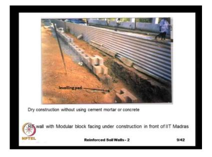
And this particular wall that was built right opposite to the IIT Madras campus, in the 1996-97 period, this was built using modular concrete blocks and these are so small that each of these blocks weighs only some 25 to 30 Kg's. And they can be handled very easily and this particular wall was constructed as part of a an approach road for a road
