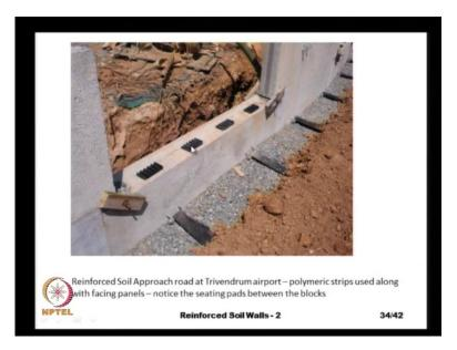
And here is another example of a retaining wall, but this particular retaining wall was built using polymeric strips, this polymeric strips are 60 mm wide and the length that depends on the on the design based on the design. We decide the length and they are connected to the front facing by using a once again, the same concept as the previous wall that we had seen with the with the steel mesh.
