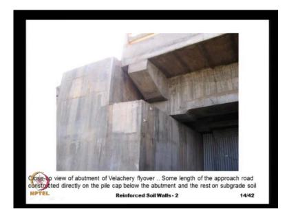
And so this is the close up of the this bridge abetment and because of the soft soil the bridge abetment was supported on number of piles and; obviously, when we have the piles we have a pile cap large pile cap.
