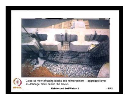
Even these modular blocks they can be used without any reinforcement layers for short height, because there is a good bonding between the different blocks through the sheer key that comes in between, well actually I do not see it here, but I will show it to you in some other lecture later on.
