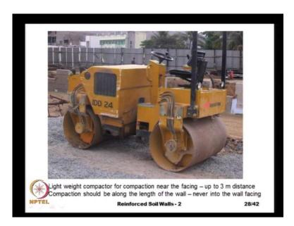
And here is a picture of a light roller half a ton roller the compaction of the soil should be done carefully, normally we try to achieve about 95 to 98 percent compaction of the back fill soil. So, that any future settlements will be very negligible or minimal, but then during the construction the facing panels, they do not have adequate support, because we are react to place the reinforcement layers.
