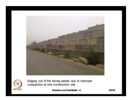
And here we see an example of that type of damage that has happened, because of the compaction into the wall, and here in this particular case this wall was built near Delhi. And here we see these two rows of panels that are bulging out and we can see the we can see the curvature is actually also indicated that through this dark line just for visual purpose.
