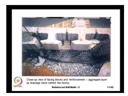
And here we see a close up of the same thing of these modular blocks, and then we see these reinforcement layer and then the aggregate.
