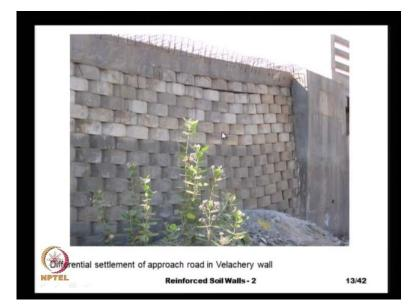
And is actually this construction of this approach road took place in an extremely soft clay and they did not do any ground improvement at the side, so there were quite a lot of settlements. And if the entire length of the wall was uniformly supported on the foundations all their would not have been no noticeable deformations, but here the then this is the reinforce concrete bridge abetment.
