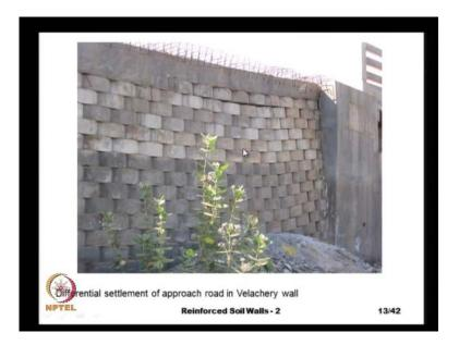
And that has led to some problem in the reinforced soil fill, so there were some cracks in the in this modular blocks, and this some difference in the alignment of these blocks, but nothing has happened to the soil itself. Because, the soil is stabilized not because of the blocks, but because of the horizontal layers of the reinforcement that we place in the soil and these the facing is mainly given for aesthetic purpose and to prevent any soil erosion.
