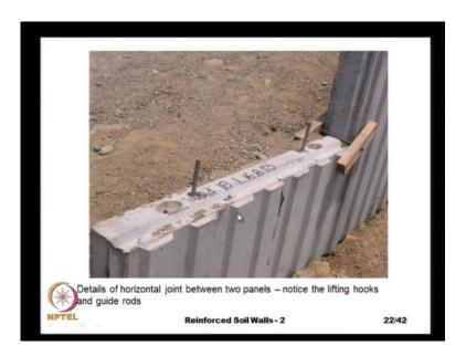
And here we see the close up of these panels and because these panels need to be handled by a crane we need some hooks lifting hooks, and here we see one hook here and then another hook here and the we need some guide rods. So, that these panels are aligned properly and then there is some bonding between the different panels, and here we see these guide rods that are pre cast in these in these blocks. And you can see the date that is 16 August 2003, that was cast in 2003 August.
