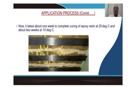
So, after you complete this, then you allow these to cure. Normally, it takes about a week time for temperature at around 20 degrees centigrade. So, let us say in an ambient temperature from around 20-22 degrees centigrade, in a week's time you expect this to get cured and achieved the strength.
