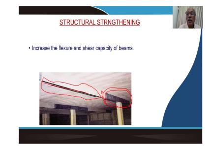
To increase the flexure and shear capacity of beams, we can use simultaneously if you see in a beam unit to increase both the flexural action as well as the shearing action. So, what do you need to do is both at the central zone as well as on the support zone you need to provide a FRP. Now, as you can see in this particular figure here.
