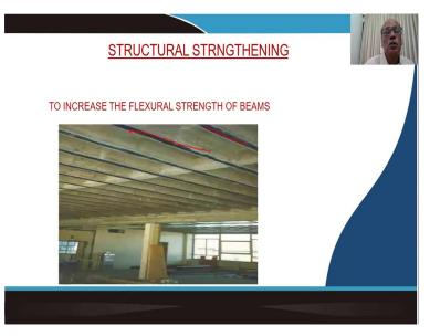
Now, this is a kind of a repairing technique that has been shown that you have a series of beams to carry the load. And as you can see over here, that soffit of the beam a FRP material has been used at the soffit of the beam FRP the material and it is been used to enhance the carrying capacity of the beams in flexural actions.
