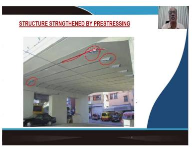
So, here I have shown you a figure where you see this the anchorage has been fixed on to the slab surfaces and the anchorage cable has been taken through this anchorage, I mean, the pretension cable has been taken through this anchorage which can be pulled on both sides, we have fixed this anchorage and then you can pull it. So, eventually it will apply a force onto the surface which is on the reverse direction and thereby will have stresses induced into the structural member.
