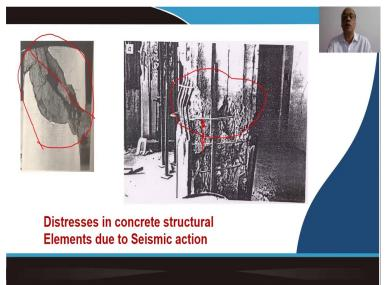
This is another example. We were talking about the earthquake actions or the seismic actions. Because of that you get lateral load in the structural system, and which can cause damage to structures. And as you can see over here, this is actually a column member supporting a deck, and you see this is a kind of failure that has happened which is attributed as the shear failure. Because of the lateral load the concrete has tried to split up.
