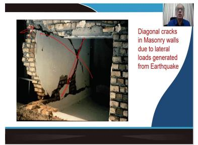
Secondly, many a times you will find, when the structural system particularly, the masonry structures are subjected to some kind of lateral loading because of the environmental loading conditions, either due to earthquake or wind, now these lateral loads tries to generate some kind of diagonal tension. And as a result as you can see over here, you have the cracking in the wall in the diagonal level.
