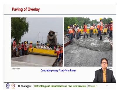
These are some of the pictures of paving of overlay. This is concreting using fixed form paver. Here, near Kharagpur, this overlay has been constructed very recently. And these are the pictures of that project IIT Kharagpur. In IIT Kharagpur that has been done. So, this is the fixed form paver and this is the transit mixture through which the concrete is poured.
