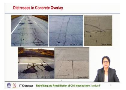
So, these are some of the pictures of distresses in concrete overlay. Here we can see that corner cracking, the concrete overlay or whitetopping is suffered from several corner cracks at these locations we can see very clearly that corners are getting damaged and corners are the location of maximum stresses. So, if the stress is more than the flexural strength, then the cracking may occur at the corners.
