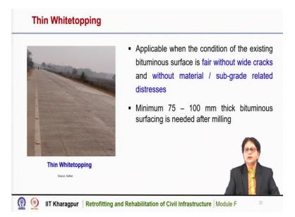
This is a typical picture of thin white topping road that is constructed near IIT Kharagpur in recent years. So, this is a typical thin white topping road, the joint spacing is much small and the panel size is 1 metre  $\times$  1 metre. Thin white topping is applicable when the condition of the existing bituminous surface is fair without wide cracks and without material or subgrade related distresses.
