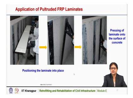
These laminates are pultruded laminates and you can see here that these are the laminates which are to be placed on the existing surface, which has been prepared for taking this FRP laminates. So, here are the positioning of the laminates into the surface at proper place. So, these are the laminates of desired width and length and they are placed with epoxy resin.
