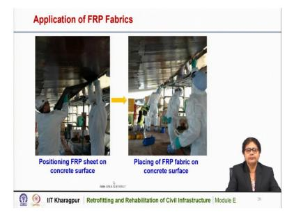
These are the pictures of the placement of the FRP sheet and fabric on the concrete surface. We can see the positioning of the FRP sheet onto the concrete surface. This is the surface where the FRP sheet is to be placed and here the placing of the FRP fabric on the concrete surface. So, these are carbon fiber fabric, that are used here for application on this existing concrete surface.
