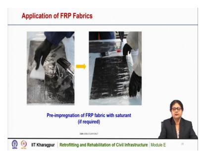
And then we can impregnate the FRP fabric with saturants. Sometimes we require this preimpregnation of the FRP fabric with saturant prior to put it on the existing surface. So, here that has been done. This is the FRP fabric and the resin is put onto it and this is the fabric with saturant.
