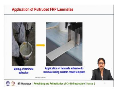
These are the pictures of application of pultruded FRP laminates. Here is the mixing of the laminate adhesive. So, the adhesive is mixed, the epoxy resin that is mixed here and then it is
