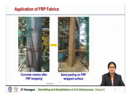
These are some of the pictures. This is a concrete column, a circular column, after FRP wrapping. This is a water tank being retrofitted with FRP. These are carbon fiber composites and this column has been retrofitted with FRP wrapping. So, just after wrapping is over, the photograph has been taken from a site in Kolkata and after the placement of the FRP composite, sand pasting is done on the wrapped surface.
