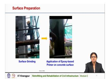
These are some of the pictures of the installation of FRP on actual structures. We can see here that surface grinding is done. This is the surface is prepared and that is done by grinding. So, here, we can see that this is an existing structure. The surface is prepared and it is made uniform and flat using grinding. And after that, it is the application of epoxy-based primer on the concrete surface. So, this is the surface it has been grinded and then the epoxy-based primer is applied.
