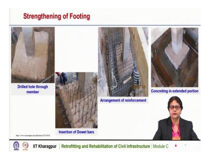
These are some of the pictures of strengthening of footing with enlarged section. We can see here that in this case the existing footing there are holes drilled through the member and through that whole, dowel bars are inserted. So, we can use also a smaller number of bars as per the requirement and then the reinforcement to be arranged.
