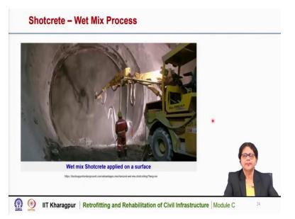
And this is a picture of wet mix shotcreting applied on the surface. You can see here this is a surface a typical concrete surface and the surface is damaged. So, to restore the surface, we can use the wet mix process.
