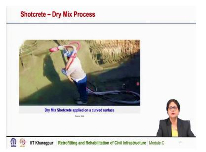
So, here is one picture, that dry mix shotcrete applied on a curved surface, you can see here no formwork is required and the mixing material is applied with high pressure onto the surface and the surface is prepared. So, this is dry mix shotcreting.
