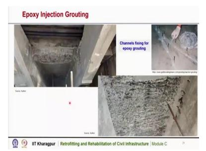
Here are some pictures of the epoxy grouting injection. We can see here, that this is a road over bridge, which is under retrofitting and the deck slab has several cracks on it. And these are the portions, which is to be grouted with epoxy injection. Small ports, or channels, are placed on the surface and through which the epoxy grouting can be done.
