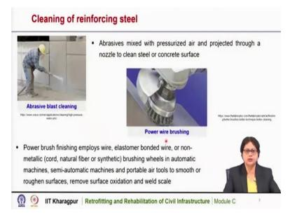
We can also use abrasive blast cleaning technique, or power brushing, by which we can remove the rust over a reinforcement steel. Now, in abrasive blast cleaning the abrasives are mixed with pressurized air and are projected through a nozzle to clean the surface. You can see here the it is applied through a nozzle with high pressure and the surface is cleaned.
