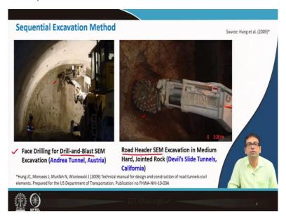
So, now you can see that the sequential excavation is going on. What is written first one is the Face Drilling for Drill and Blast SEM. So, you can see that drilling is going on. On the other hand, roadheader SEM excavation is performed in medium hard jointed rock.
