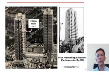
You see on your screen the Ronan Point buildings these were 22-story tall apartment buildings in East London completed in 1968 with 5 apartments per floor they promised efficient and affordable urban housing. It was a precast construction rather new at that time and chosen due to ease and speed of construction. So, every element the walls the floors the staircases they were precast and each floor was supported directly by the walls in the lower stores.
