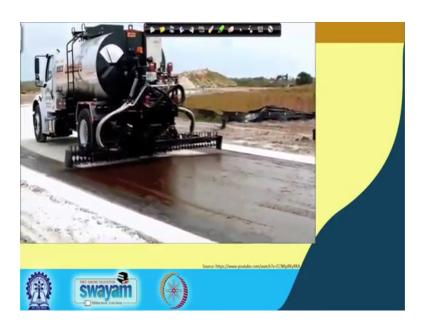
Plastic roads the laying procedure: the laying procedure for the plastic roads will be the same from the subgrade course to the base course like any flexible pavement.
