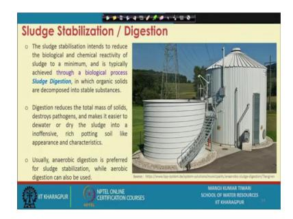
So, we will begin with the sludge stabilization. Stabilization essentially the digestion process slow sludge is stabilized intent which is kind of idea is to reduce the biological and chemical reactivity of the sludge. Then what we call it to be like a stabilized sludge, when there is not of not much of biological or chemical reactions taking place within the sludge zone, or within the sludge medium. And this is typically achieved through biological processes which is called Sludge Digestion.
