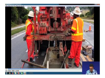
So, as I mentioned. So, you can you can increase the depth of these or the height of the drill rod by adding one after another. So, we can go up to the required depth.
