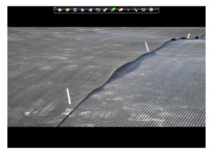
This is the Geonet material, especially it is used for the double liner system. Do not worry too much about this but for the hazardous waste it is used. This particular MSW landfill which was in a very close to certain environmentally sensitive area, so they actually went ahead and did a double liner system here.
