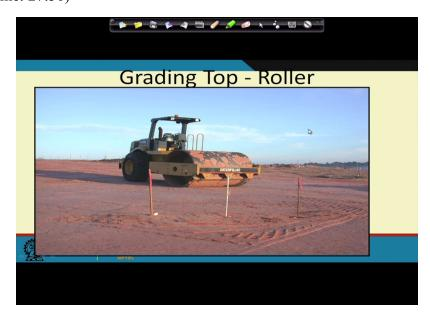
So to avoid that, what we will do? Very simple, we put a thin layer of clay on top. So just make a nice layer on top as you can see in this particular picture, it is a nice layer of clay and then after that you do a grading top and pass through a roller. Very similar to roller that you see on your
