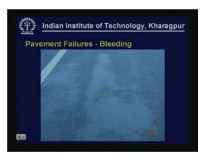
Another failure that is more or less related to rutting or caused because of similar reasons such as bleeding which is the occurrence or presence of excessive bitumen film at the surface. Though it's not a major structural failure but this reduces the skid resistance of the pavement surface and also it does not give a good impression of the pavement that is constructed.
