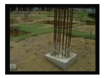
So, detailing also it is not the unique solution you can have number of solutions also. And this is you say 1 circular column and with spiral that not only we can provide ties, but also you can provide that 1 say spiral binding like this we can go. So, when you come to this 1 these are the different components that we have to provide, in addition to that we have when you consider these all of them.
