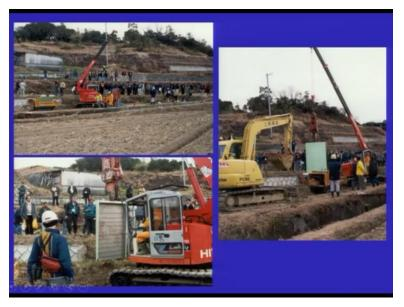
So this is an exercise, which is commonly done in Japan, where the geoslice has been used to locate the fault trace. So here instead of opening multiple trenches, you can easily put. So for example if you identify the probably the fault running somewhere here on the surface. Then you can have multiple slices, which you can take from different location okay and that can also help you in identifying the orientation of the fault. So this is the first plate, which has been pushed into the ground.
