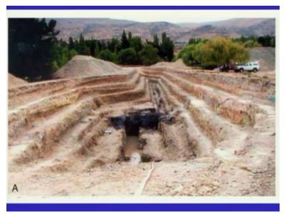
There is another way of trenching, which is very common to the opencast mining, which has been done here. So it is a very wide trench and this is more or less very safe in the sense, because you are creating steps; you are not creating the steep wall and if you are doing this type of trenching, then you can go deeper. You can reach to the deeper portion of the fault or the displaced units.
