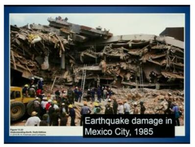
Then coming to 1985 Mexican earthquake the pattern of damage you can see so basically what we are looking is the poor construction without having an proper understanding that what will be the amount of or the intensity of ground shaking by a particular earthquake in that region.
