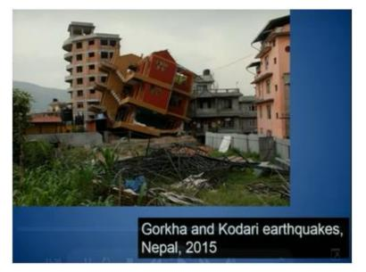
Coming to the gorkha and kodari earthquakes in Nepal 2 earthquakes took place in this region in 2015. The damage was not so severe, but of course it was bothering for us actually. So this was the building one of the school building which collapse the columns were broken because of strong ground shaking near Kathmandu.
