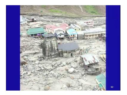
This move in this picture is here which shows that lot of big boulders which came and stopped behind this tower and was responsible for saving the whole structure, but rest of the area was completely in mess. So, damage was severe because of sudden pouring of huge amount of water due to cloud burst and which triggered in turn the debris flow.
