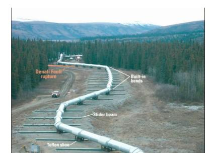
So, this is the after the earthquake photograph was taken, where you can see clearly the exact form of the pipeline which was because of the fault moment and of course also due
