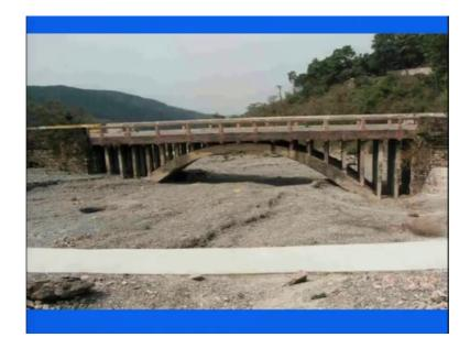
So, what they do is that periodically they keep dredging and then allow create enough cross sectional area that is allow the water to flow down. So, to stop the sediments getting filled up in this part particularly they constructed and retaining wall, but that did not work as I was I discussed in the previous lectures of when we were talking about the landslide. It broke it because of the sub surface erosion within the channel.
