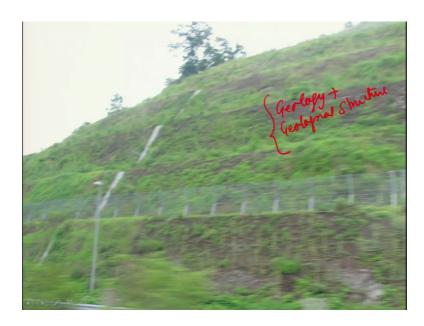
It is another example. This is from Japan whether the combination of three what they have uses one is the wire mesh here they have reduced the slope putting the benches reinforcement has also been then. And then and water pathways have been constructed to drain out the water as fast as possible. So, you can depending on the geology of the area plus the geological structures present. You can have different combinations close up of that.
