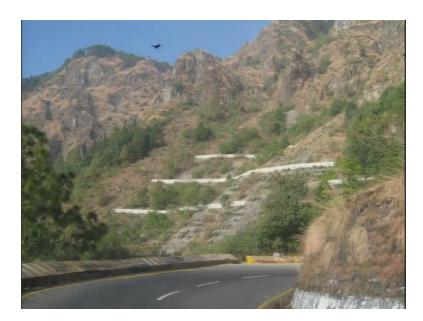
Similar thing has been done some slope angle has been reduced as well as been protected by putting the retaining walls.
