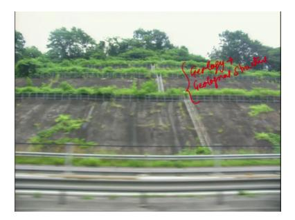
So, you have the wire mesh this is basically done for the beautification also and then you have number of drainage or the water pathways which have been consecutive to remove the water when not allowing the water to percolate down as early as possible as well as they have done the reinforcement.
