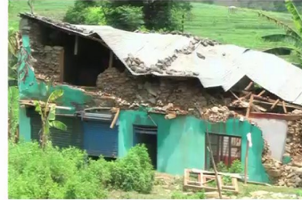
Photo 4: Collapse of first floor stone masonry packed in mud-mortar and GI sheet roof of a house at Naya Sandhu village
