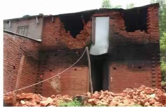
Photo 3: A brick masonry-mud mortar structure suffering damage of Grade 4 in Chebetar Village
