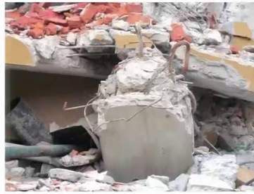
Photo 9: Failure of load bearing base column from beam junction, Thankot. Central region, Bagmati, Thankot, Tribhuvan Highway, Nepal (27°41'25.7"N; 85°13'20.7"E)
