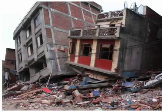
Photo 6: Collapse of RCC framed structures due to failure of load bearing base columns of the stilts in Kathmandu Valley. Central region, Bagmati, Kathmandu, Chhauni, Nepal (27°42'45.0"N; 85°16'58.5"E).
