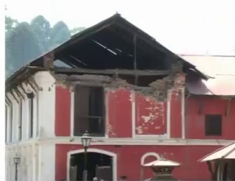
Photo 7: Collapse of brick masonry-mud mortar gable wall of a structure of the Temple Complex
