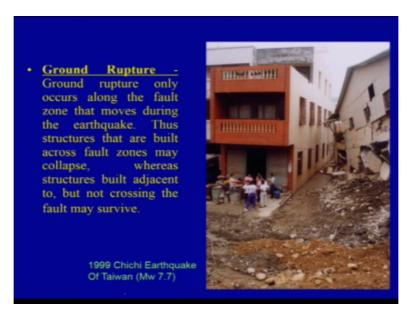
So and this is a very good example which has been given okay that the house which was sitting close to the rupture, okay that is the fault line, got damaged here but the other house just escaped the damage, okay so this is the another important part okay, fine and this is from Taiwan, during the the chichi earthquake, 1999, magnitude was 7.7.
