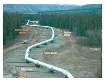
So what they did was they decided that fine let us bring the pipeline on the surface rather than putting subsurface and since they knew that this fault is a strike-slip fault a right lateral strike slip faults which will definitely will have a movement where one block will move towards right and another towards left or maybe we can say that the block will move towards us. So they knew the sense of movement and then what will be the offset.
