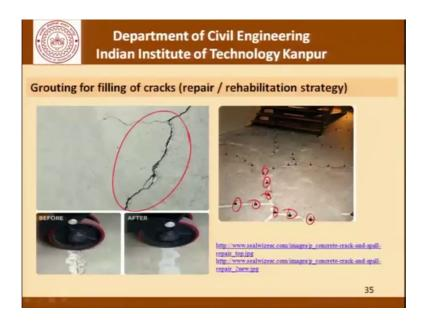
So, this is a crack in a concrete structure and we are trying to fill this up using grouting. So, these are places where successively grout is being injected and we ensure that once the grout appears in the next nozzle we tried to seal that and move forward. So, by doing that throughout the structure we achieve a complete sealing of the concrete crack.
