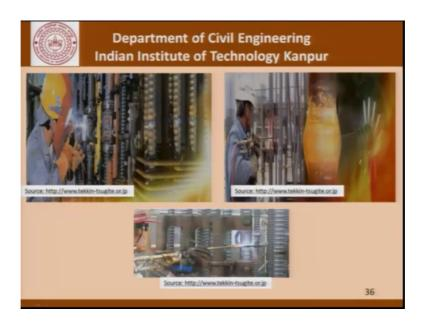
Now, these pictures here show site conditions where this gas pressure welding is been carried out. And again we see the importance of a workman the person who is actually carrying out the work it is the skill which is involved and there are 100s of bars to be welded.
