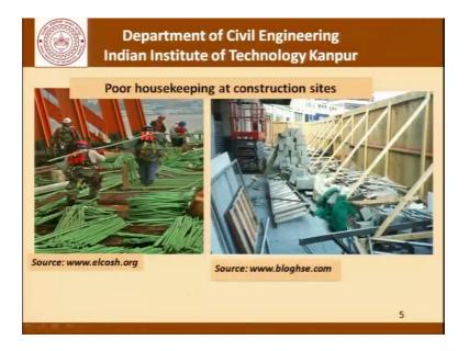
So, here are two pictures which show an extremely cluttered site and you can imagine that working in these sites is an additional challenge than working in normal environment to self. The picture on the left has bars lying all over the place and the workers have to be very careful to avoid tripping on these bars as they move carrying a bar from one place to another.
