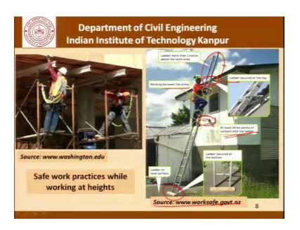
So, here we see some safe practices while working at heights with ladders and this picture here especially shows us how to handle a ladder. So, there is ladder should extend
