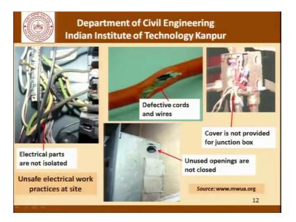
So, moving on here we see some unsafe electrical work practices at site. It could be non isolation of electrical parts, it could be defective cords and wires, it could be the cover not been provided on the junction box or it could be an unused opening which is not closed. All these becomes sources for increase in the vulnerability and susceptibility as far as accident is concerned.
