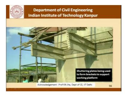
Now, let us take a look at some of the unsafe conditions and photographs from sites where we will be able to clearly see how safety norms are violated. Here for example, we see shuttering plates being used to form brackets to support platforms.
