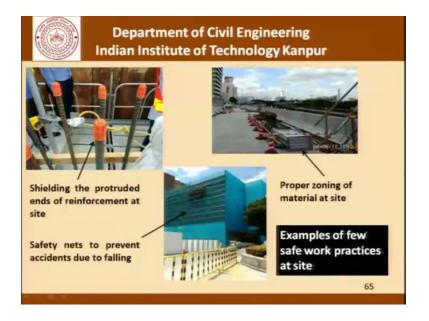
Now, after seeing so many poor housekeeping slides this is an example of a better management where there is shielding of protruding ends of reinforcement, safety nets and proper zoning of the materials at site. So, it is not that it cannot be done it is only a matter of having the will to actually do it.
