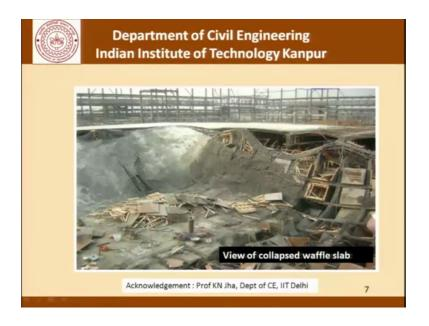
This is another accident where we can see the collapse of a waffle slab. So, we can see that once an accident happens there is so much of reconstruction that has to be done, there is so much of loss that has happened that it is very very difficult to recover from that. The cost of an accident is simply very high those are things which we need to talk about and at least be aware of as construction professionals.
