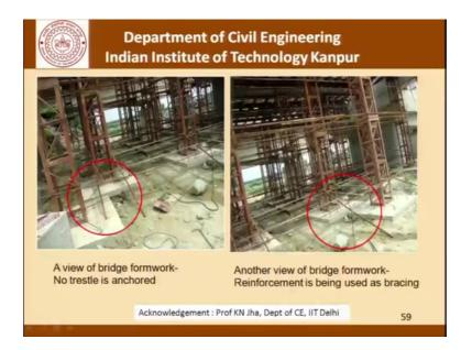
This is the view of a bridge formwork with trestles not anchored and another view where the bridge formwork reinforcement being used as bracings. It is important to understand that no matter what the worker does the management must ensure a clean site it is important for the execution team to have good housekeeping and good practices being practiced at site and therefore, such conditions are unsafe conditions arising out of misuse of tools misuse of material and so on.
