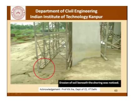
We find shoring where there is erosion of soil beneath.
