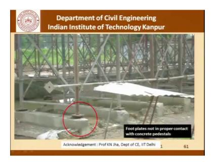
Here we find foot plates not in proper contact with concrete pedestals.
