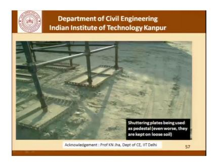
Here we see shuttering plates being used as pedestals and even worse they are kept on loose soil.
