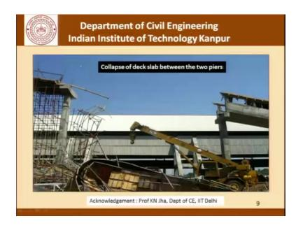
This is a view of a collapsed deck slab between two piers.
