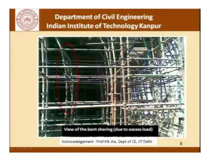
This picture here shows bent shoring, now this bent shoring could be on account of excessive loading.
