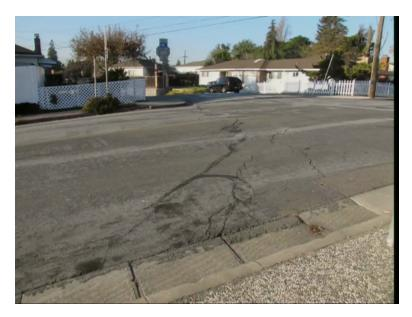
And then another photograph close up of that ok, so you can see here the cracks which are coming up on the on the road ok, so fault runs through here ok, goes here so this is the zone here ok and close up of this let us see close up of this one ok.
