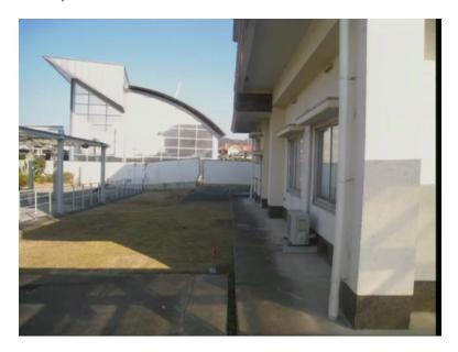
Close up of that house and the wall which you can see here, so fault just crossed this one here, this side is up, this is down and with some lateral displacement.
