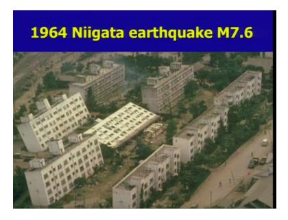
There is an example 1964 Niigata earthquake. The building were toppled down because of the loss of shear strength of the underground material so this is again an example of liquefaction okay. So if the land lost the shear strength or the surface lost the shear strength because of strong seismic shaking which was resulted by liquefaction.
