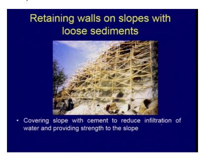
Then our example of retaining walls, you can do and cover the slope with cement and reduce the infiltration and also strengthen the the slope.
