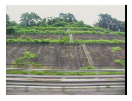
So again this is the example of the drainage which is coming up and they have reinforced, they have put concrete on the surface to protect that and at various locations where they have cut and reduce the slope, they have put such wire meshes.
