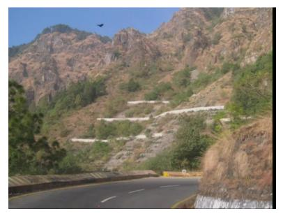
So massive landslides, you will be, you will across in the areas so this is what they have done. They have constructed the retaining walls and they have tried to reduce the slope here because this is the massive landslide which has been seen on the way.
