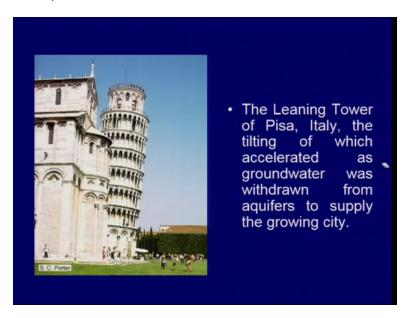
And this is one of the famous example because of the excess extraction of the groundwater okay. This is leaning tower of Pisa in Italy and this was because of the groundwater withdrawn okay so we need water for the growing cities but we may experience or we may result into the associated hazard because of this.
