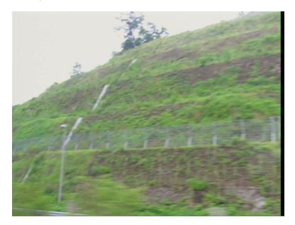
There is an example from Japan where you can see the, I may be having better photograph or not, may be this one okay so you have the drain which is coming up down here okay and then you have, they have cut the slope in different benches so they have reduced the slope here and they have tried to stabilize and in some places, they have also put the fences here okay or the the wire mesh too. If if something happens and if some block roll downs, it will be blocked here okay.
