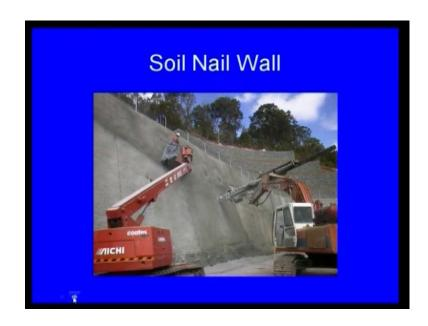
Then soil nailing wall, if you look at this soil nailing wall; these are all reinforced wall you can say it will look at this soil nailing wall this is your slope along this slope the soil nail has been provided if you see this is of, then reinforce soil nail walls if you see once again soil nail wall soil nail wall this nails how this nails as been provided.
